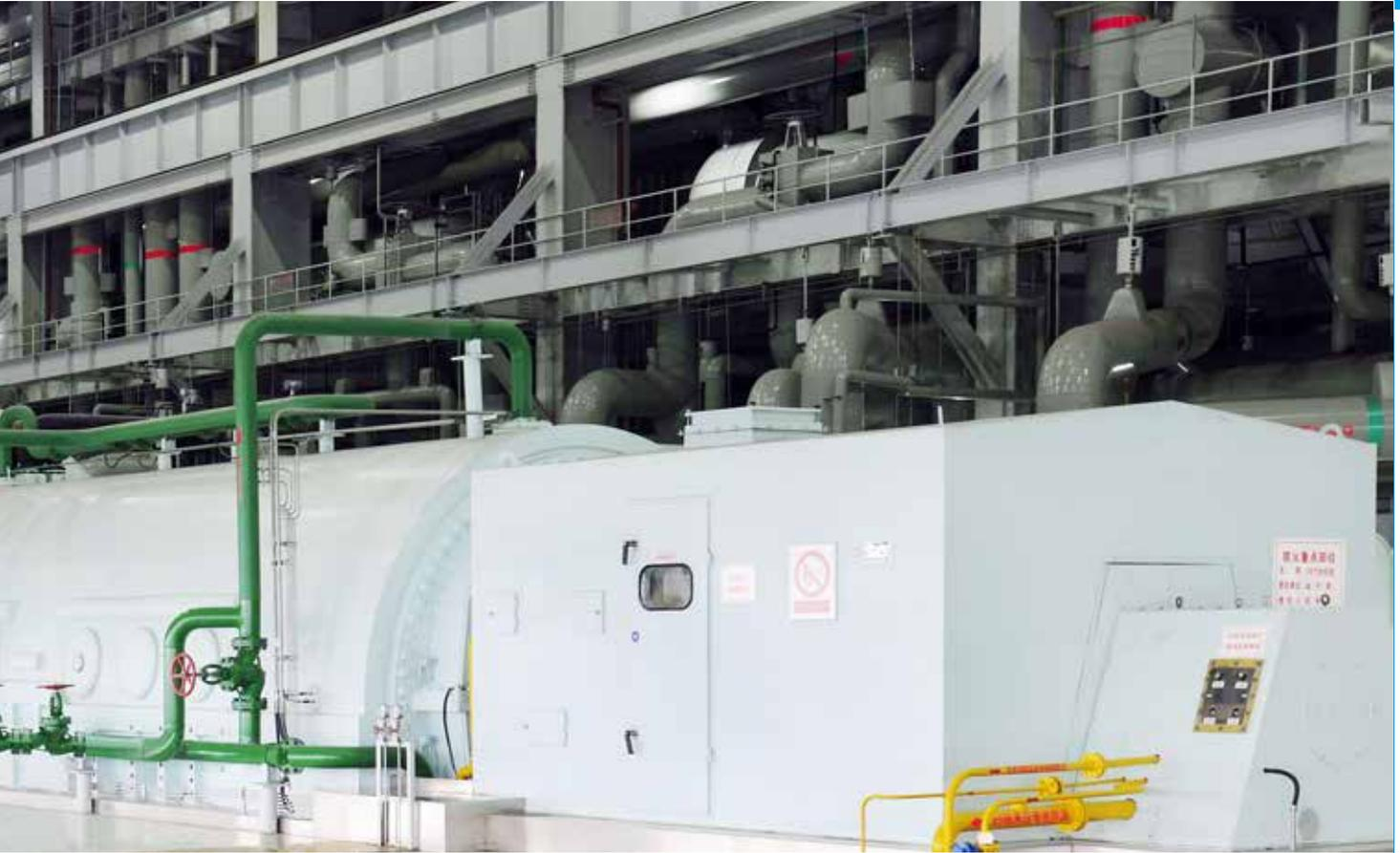
*Typical Project: The first 20MW ultra-high-speed positive-pressure explosive-proof frequency control synchronous motor in China*
